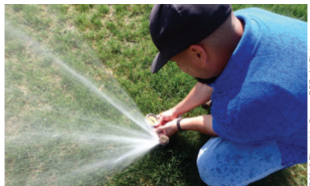
Jose Iniguez, irrigation auditor, evaluated a sprinkler system for uniform distribution of water.
